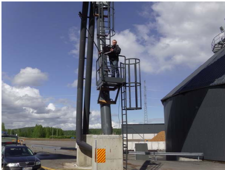
Figure 11 – The 3D-scanning were done from 5 meter high stairs at the power plant (Photo: Antti Asikainen/Luke)
