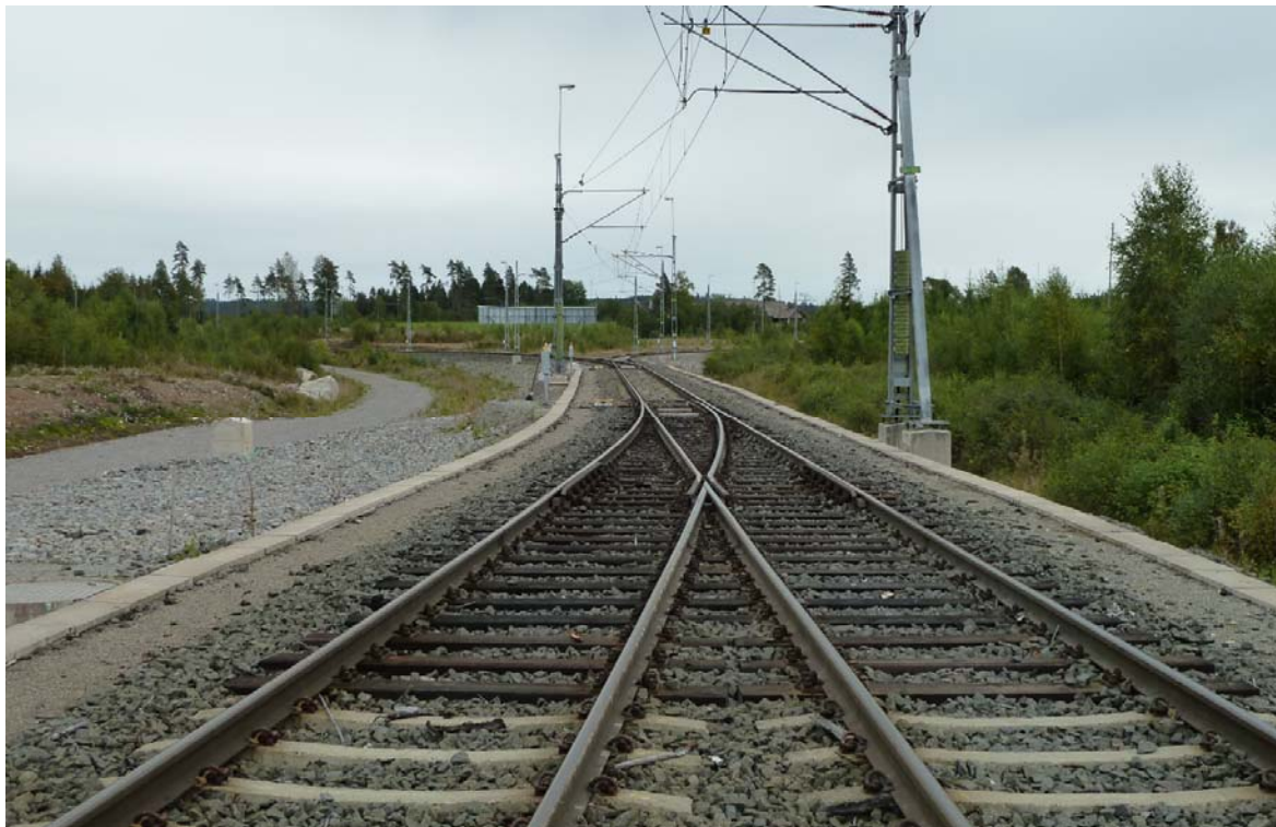
Figure 4. A triangular track connects the terminal in Stockaryd with the main track (named Södra stambanan). The picture is taken from the terminal looking in the direction of Södra stambanan. PHOTO: Stockarydsterminalen
