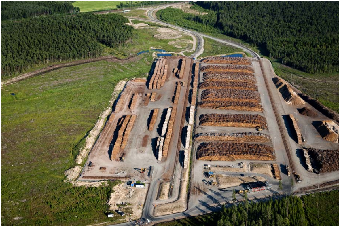
Figure 1. An overview of Stockarydsterminalen. The left track belongs to Stockarydsterminalen AB and the right to Stora Enso. The ditch in the middle separates the two parts. A triangular track is visible at the top of the photo and a measuring station that is used to measure incoming materials is seen at the bottom. PHOTO: Stockarydsterminalen AB.
