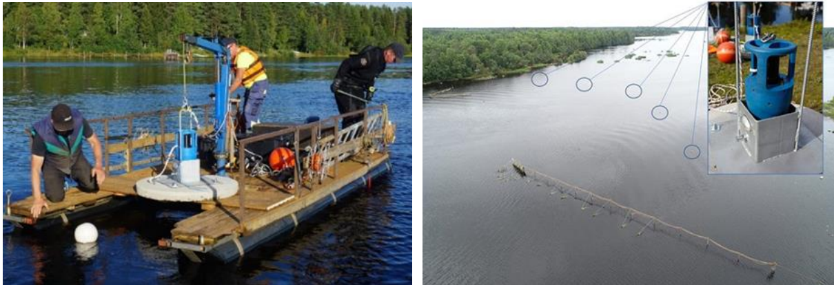
Figure 6. Left: Lowering a deterrent on a concrete weight into the Iijoki River. Photo: Petri Suuronen. Right: Five deterrents placed in a line across the main channel. The fence of a fish weir near the deterrents is visible in the foreground. Photo: Lari Veneranta
