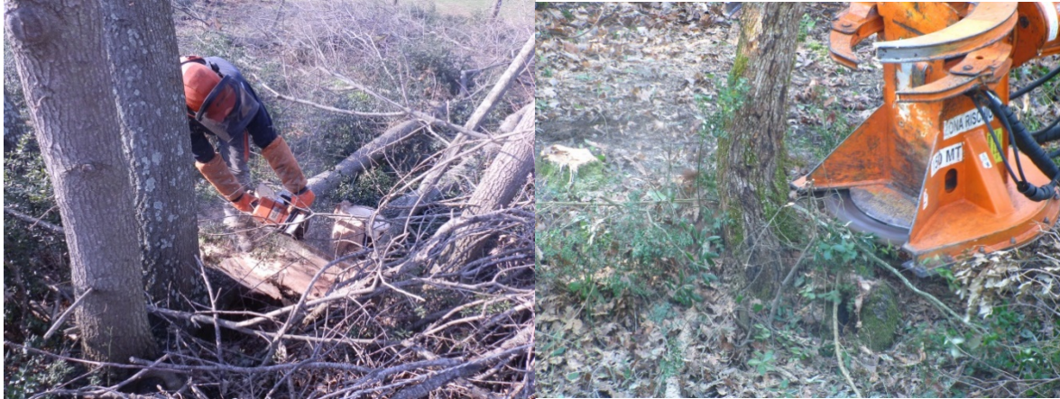
Figure 6. Cutting by chainsaw (left) and by disc-saw (right).
