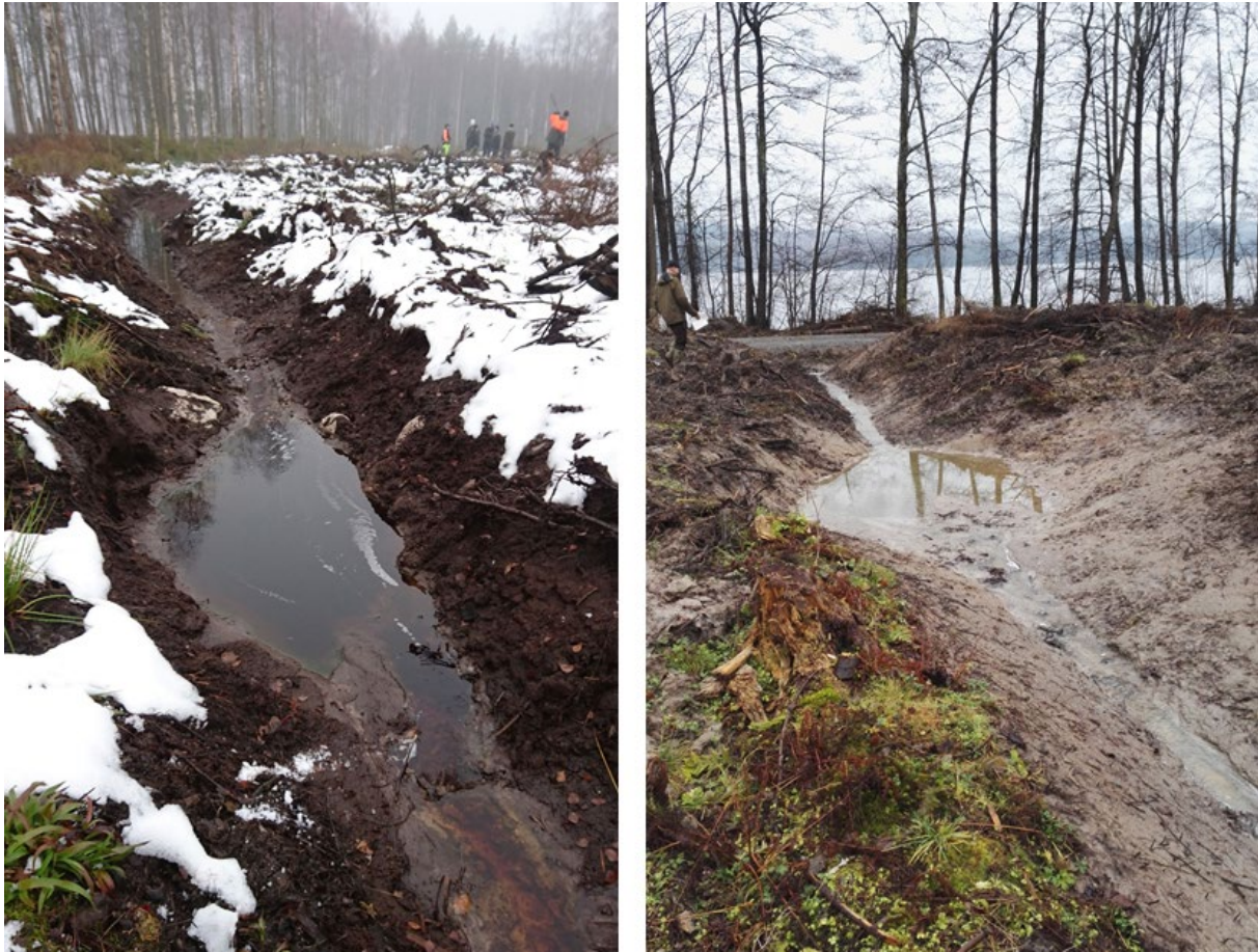
Figure 4. Sedimentation pits in drainage ditches in southern Sweden. Photos by Eva Ring (left) and by Anja Lomander (right).
