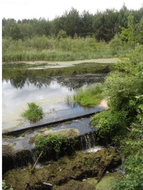
Figure 32. A gabion sill for outflow of water from a reservoir in Poland. Photo by Edward Pierzgański.
