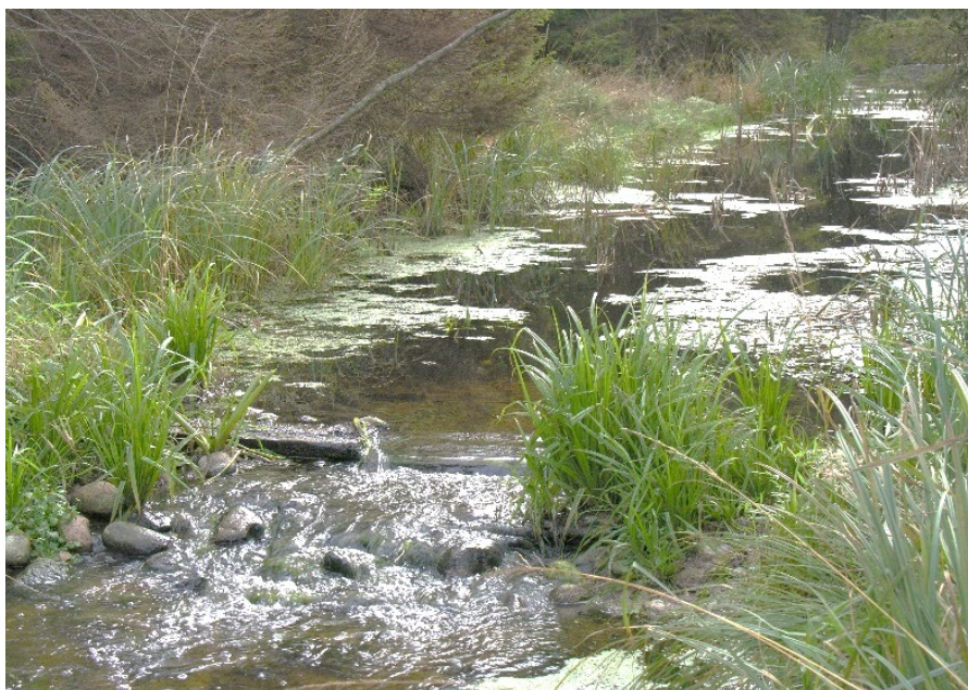
Figure 24. A sill constructed from wood. Photo by Andrzej Ryś.
