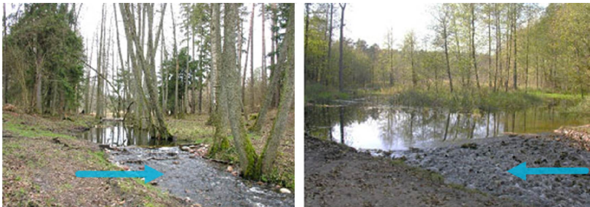
Figure 26. Sills with fish passes belonging to the “close-to-nature types” and called as bottom ramp and slope. Their sill has a rough surface and extends over the entire river width with as shallow slope as possible, to overcome a level difference of the river bottom (FAO.2002). Photo by Andrzej Ryś.
