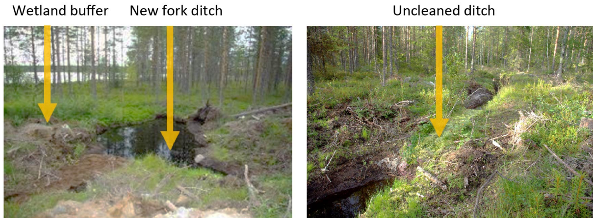
Figure 16. A new ditch dug in the form of a fork (Y) in order to distribute water to a wetland buffer in Finland (left), and an uncleaned part of a ditch (right). Photos by Eva Ring.
