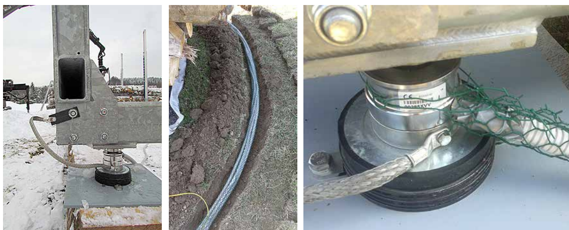
Figure 4: Earthing of the frames to protect the load cells from lightning strike (left). Cables buried in the ground to prevent temperature effects on the measurement accuracy (middle). Metal net to protect the cables from rodent biting (right). Source: Gernot Erber.
