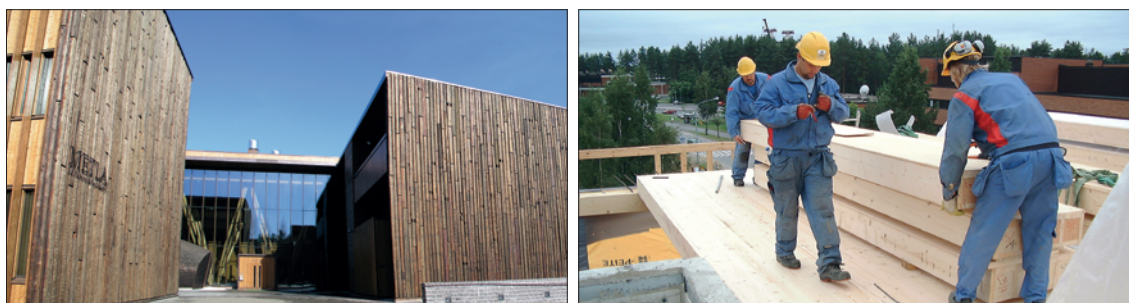
The total volume of 2000 m 3 timber utilized in the construction of Metla House in Joensuu (left), the first largest office building in Finland, provides the carbon sequestration capacity that together with substitution during the life time corresponds to 1460 tons CO 2 eq. Using wood as construction material for the Metla House has saved 620 tons of CO 2 compared to an analogous concrete solution. (Vatanen 2005) Installation of the timber intermediate floor elements at Metla House (right). Photos: left Metla/Erkki Oksanen, right Onni Miettinen
