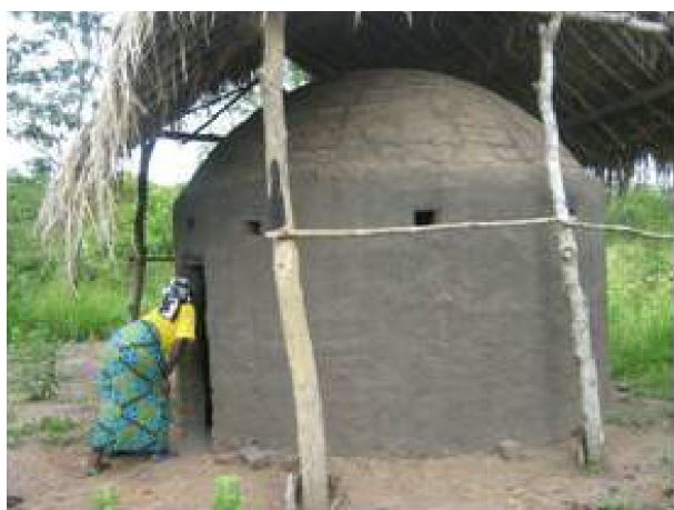
Figure 3. Half Orange Kiln at Mazizi, Morogoro, Tanzania.
