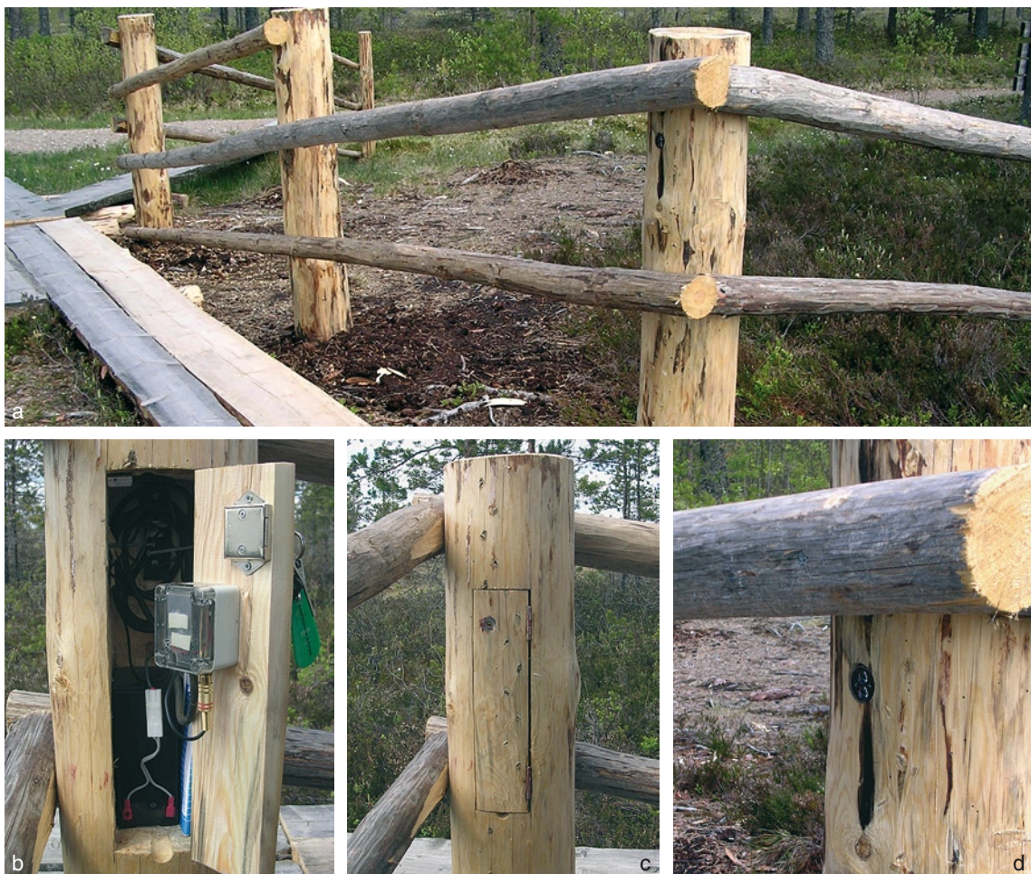
Figure 3.7 a-d. Installation of electronic counter in a wilderness area in Finland. (Photographs provided courtesy of Rami Tuominiemi)
