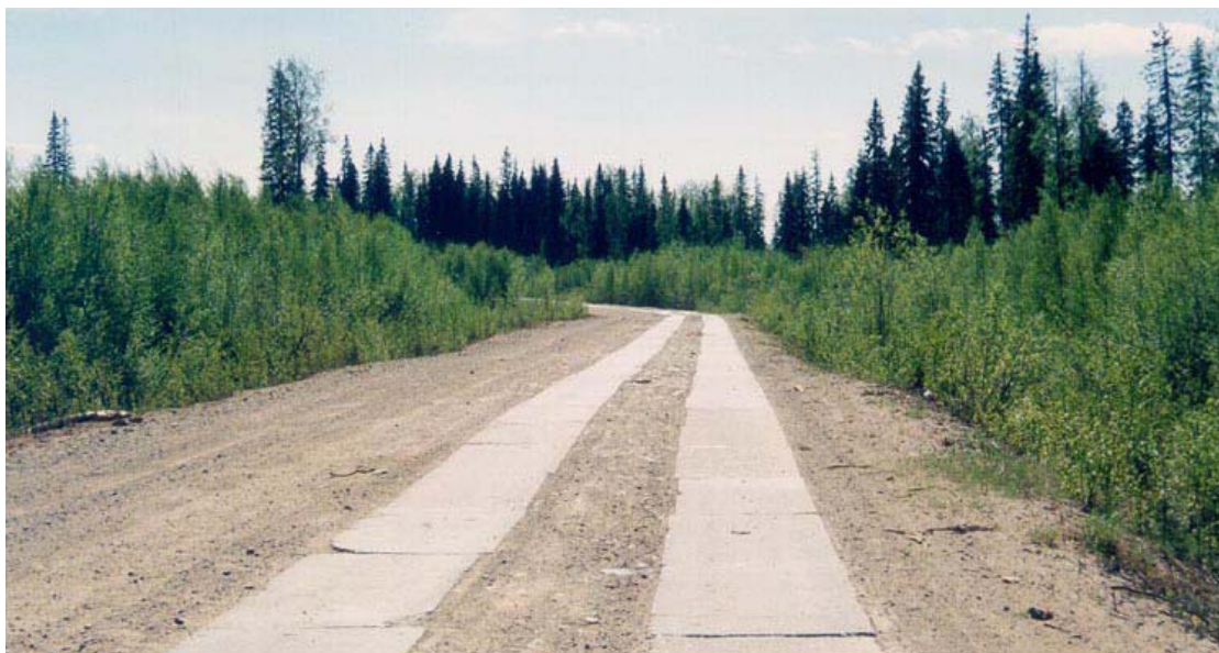
Figure 28. Betony-paving is used in areas where local rock material is not available for road construction. (Timo Leinonen)
