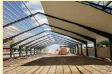
Construction of a new cowshed in the Jönköping region.
