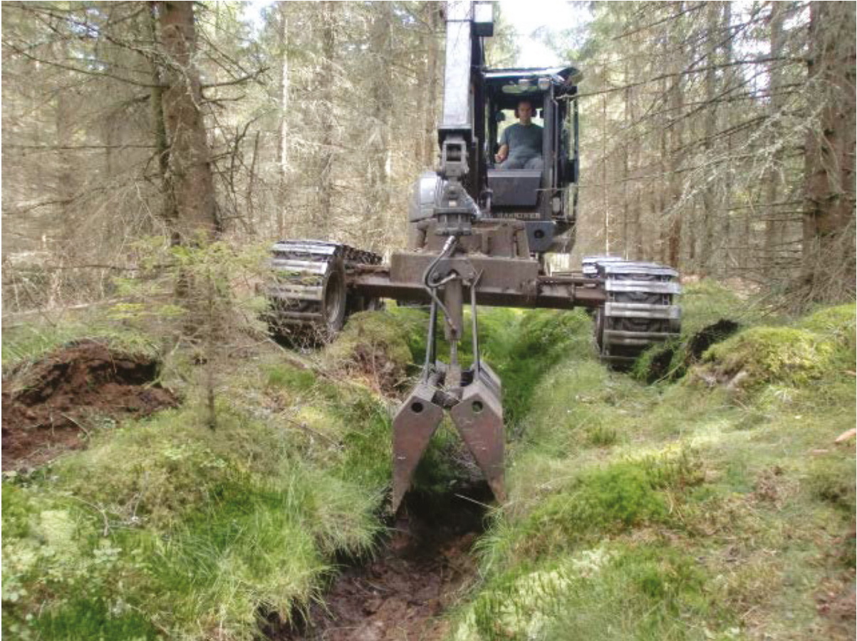
Photo 5. A ditch-bottom cleaning machine (called Varanen) doing ditch network maintenance in southern Sweden. To date there are no studies of its impacts on erosion and how long-lived the ditches are after cleaning. Photo Anja Lomander.
