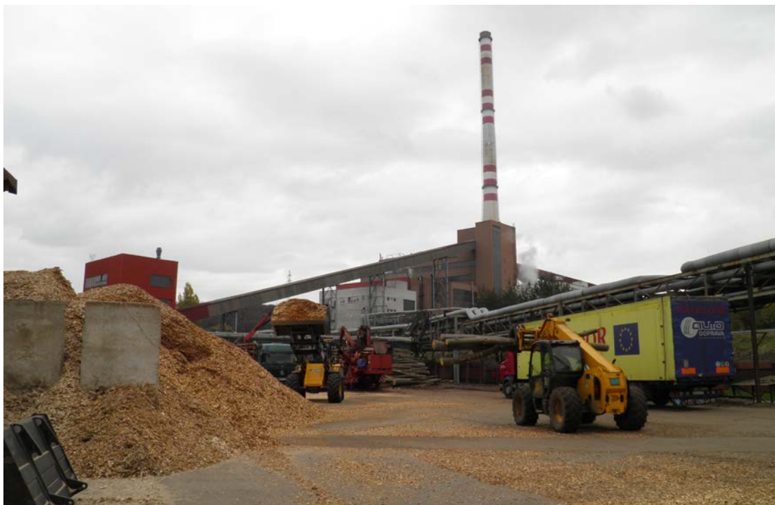
Figure 31. Combined heat and power plant in Zvolen (Source: Otepka, 2013).
