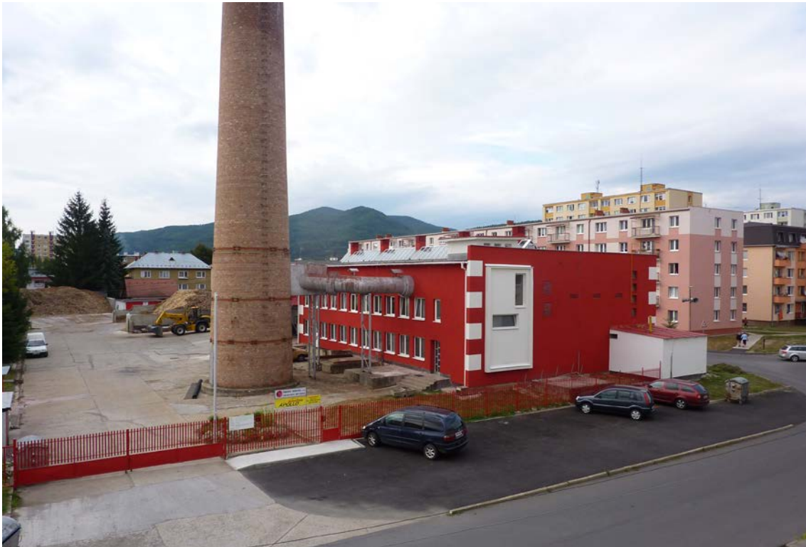
Figure 35. View of the Žarnovica heating plant (Source: INTECH, Slovakia).
