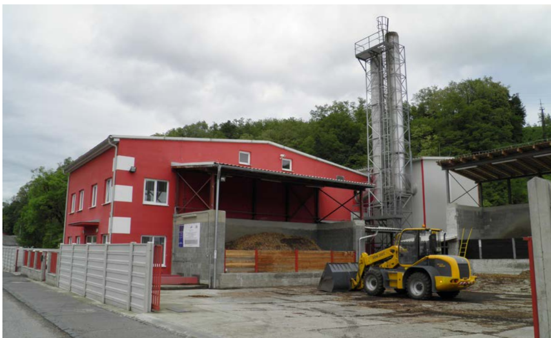
Figure 33. View of the Hnúšťa heating plant with a fuel storage place and a boiler house (Source: INTECH, Slovakia).
