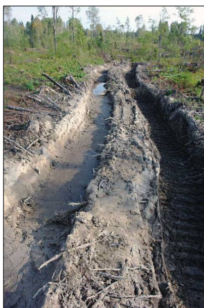
Fig. 3.13. A main strip-road track formed after multiple forwarder trips
