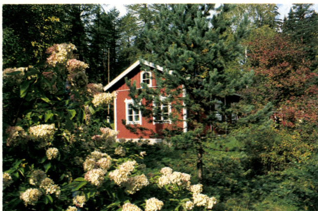
The renovated office of the Finnish Forest Research Institute.
