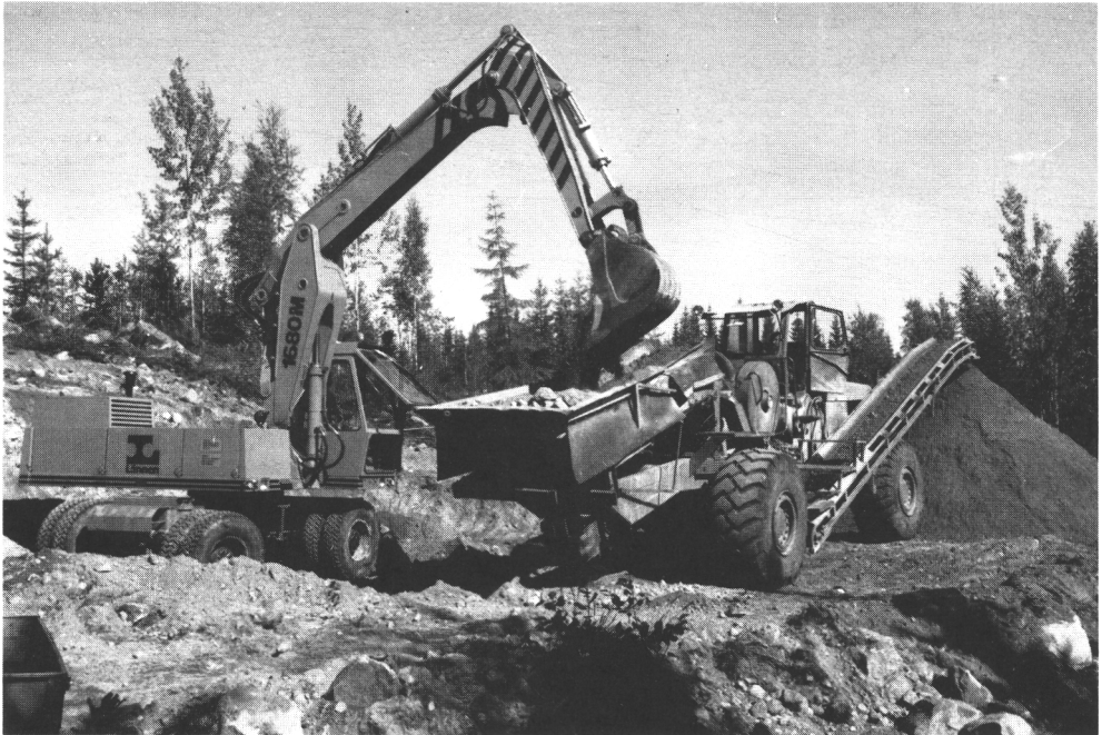
Fig. 1. The Mertsä mobile moraine crusher working at an old gravel pit. A Lännen 1680 M excavator is feeding the crusher.
